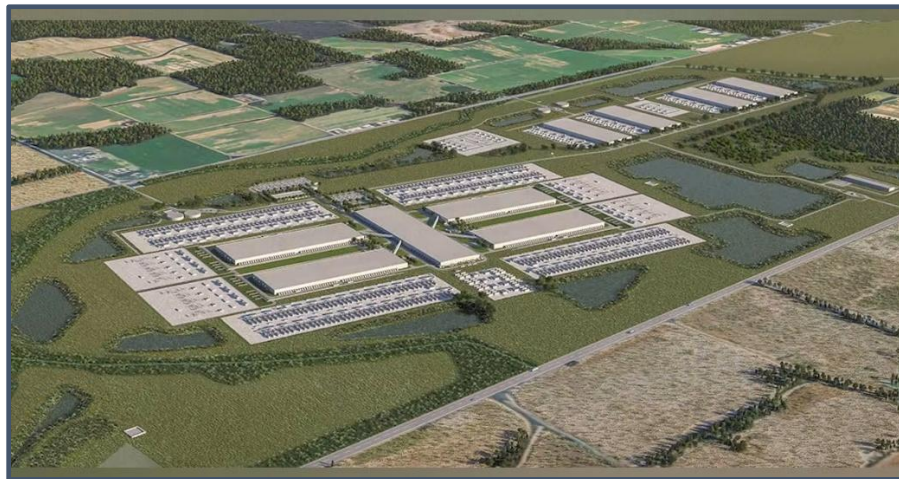
Meta's Hyperion Data Center-Richland Parish, Louisiana
